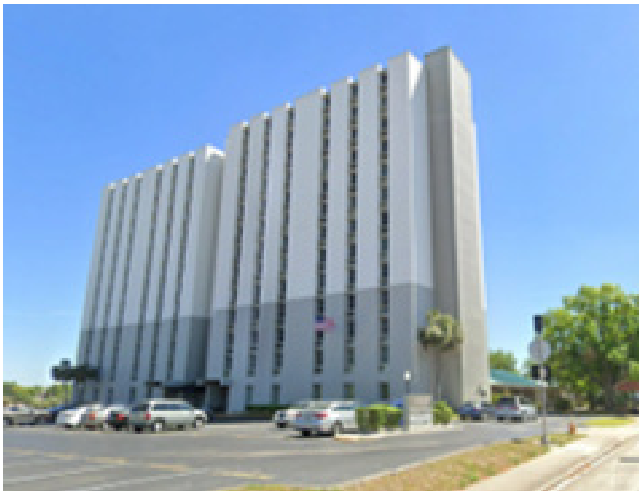
Existing Tall Building
